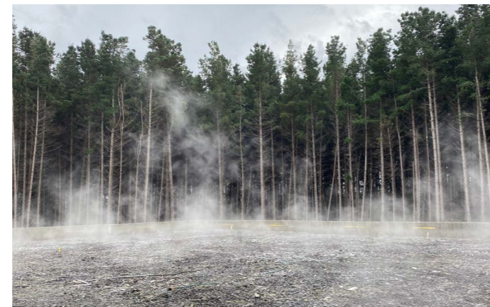
Photo. Biological odour treatment system, BioMar Australia
